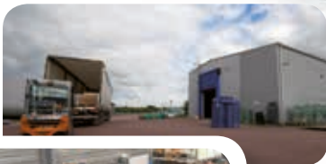
A 4 hectares storage area Tests area and logistic solutions
